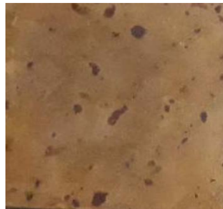
Fig. 9. Mud concrete floor final product
