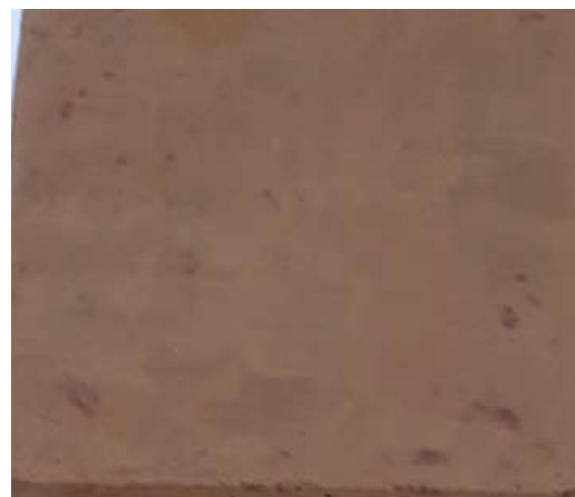
Fig. 5. Prepared floor samples for application of top surface layer after applying clay plaster
