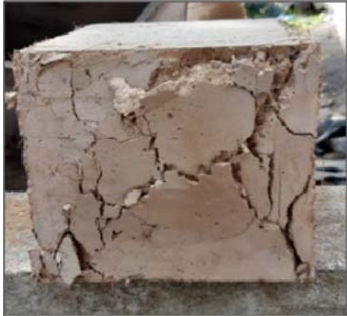
Fig. 7. Failure pattern of fiber reinforced mud concrete
